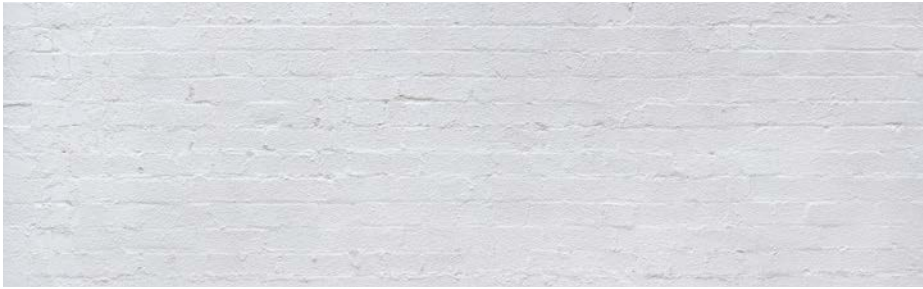
V14T58 Painted Brick Wall
