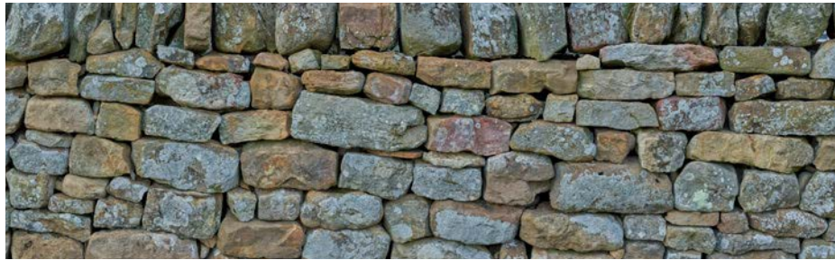
V14T51 Dry Stone Wall
