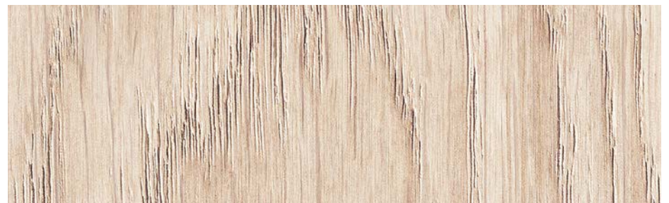
Closeup at 3m high
